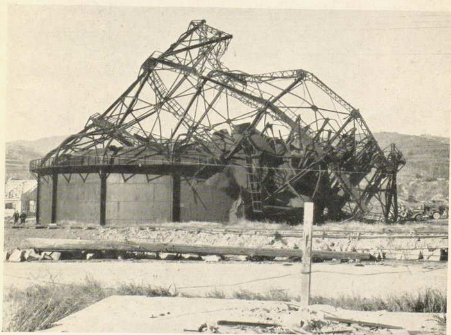
Photo No. 14. NAGASAKI. Blast effect on a gasholder \frac{1}{2} mile from centre of damage. Note the way in which the whole framework has been bent away from the explosion. See paragraph 43.
