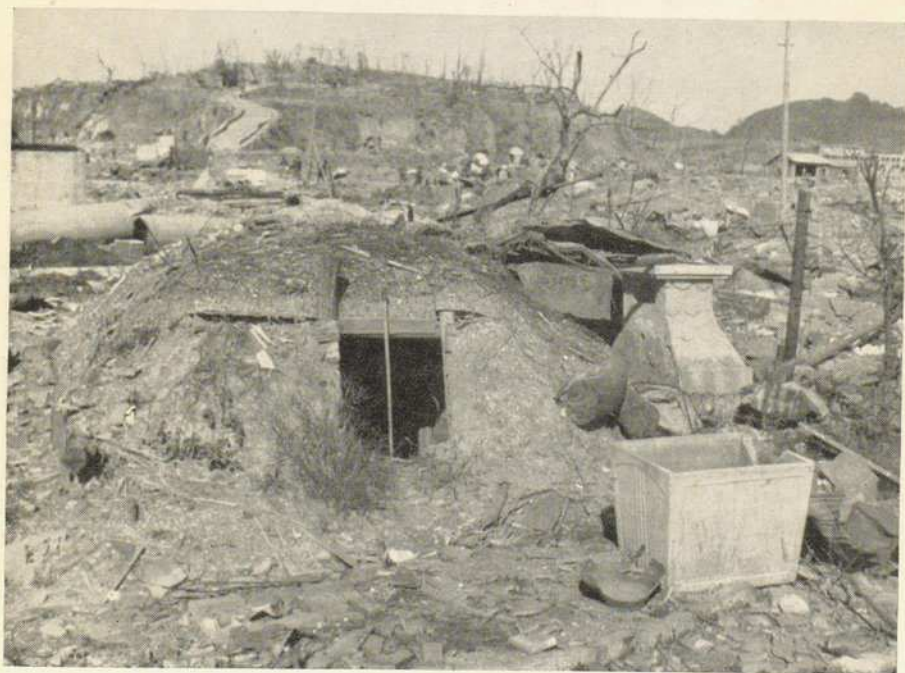
Photo No. 18. NAGASAKI. Typical small earth-covered back yard shelter with crude wooden frame, less than 100 yds. from the centre of damage, which is to the right. There was a large number of such shelters, but whereas nearly all those as close as this one had their roofs forced in, only half were damaged at 300 yds., and practically none at half a mile from the centre of damage. See paragraph 41.
