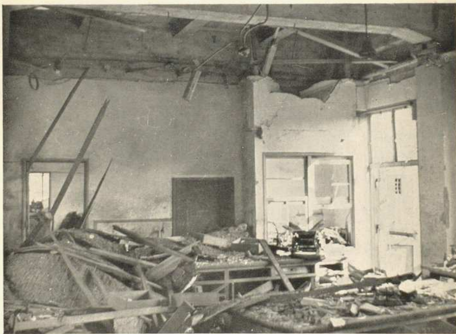
Photo No. 20. NAGASAKI. A room in the concrete hospital, \frac{1}{2} mile from the centre of damage. The building was structurally undamaged, and one of the few of its type to escape internal fire damage. The collapse of suspended ceilings, partitions, etc., caused many casualties; fire would have increased their plight. See paragraphs 68 and 80.
