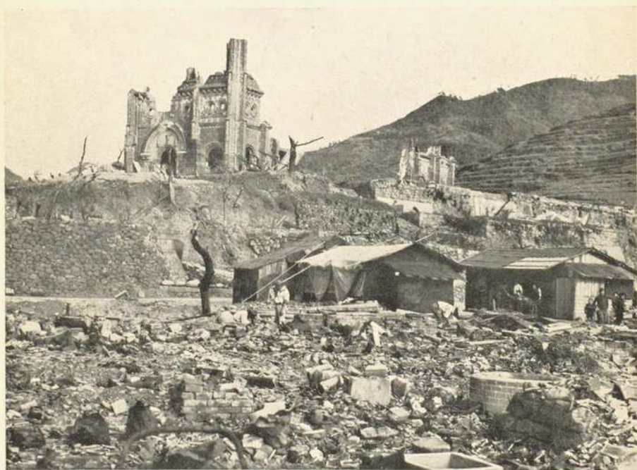
Photo No. 16. NAGASAKI. The Roman Catholic Cathedral 600 yds. from centre of damage. The walls were of heavy load-bearing brick construction. Most of the damage is attributable to blast, although fire subsequently consumed all combustible debris. Note in the foreground the huts erected by the Japanese for temporary living quarters after the atomic bomb raid. See paragraphs 11, 16 and 39.
