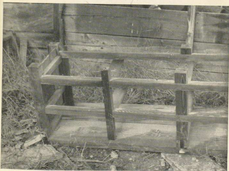
Photo No. 22. NAGASAKI. Timber framing scorched by heat radiation at \frac{3}{4} mile from the centre of damage. The surface is unscorched where it is shielded by the uprights. See paragraph 52.
