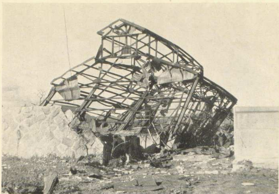
Photo No. 11. HIROSHIMA. Small steel framed shed \frac{1}{4} mile from the centre of damage, showing the distortion of the entire framework, with the building leaning away from the explosion. See paragraphs 22 and 32.
